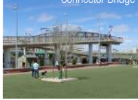
City of Philadelphia Schuylkill River Parks Connector Bridge
