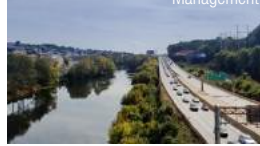
PennDOT 6-0 I-76 Integrated Corridor Management
